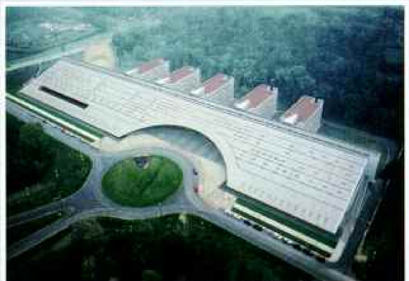
ELECTRICAL ENGINEERING SCHOOL BY DOMINIQUE PERREAU. PHOTO BY NATHAN BERRY
