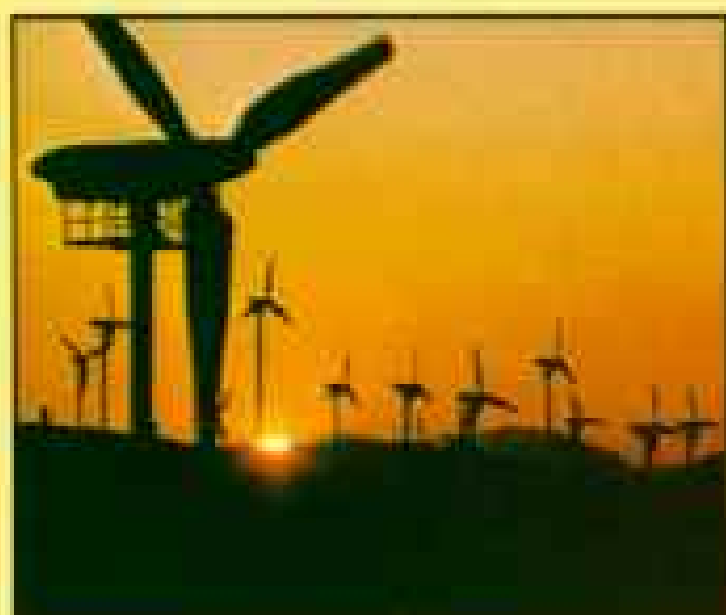
Reliability and strength of the wind play an important role in the location of "wind farms" like this one in Allamont Pass, east of San Francisco. Wind generators are spread over hundreds of acres of land.
