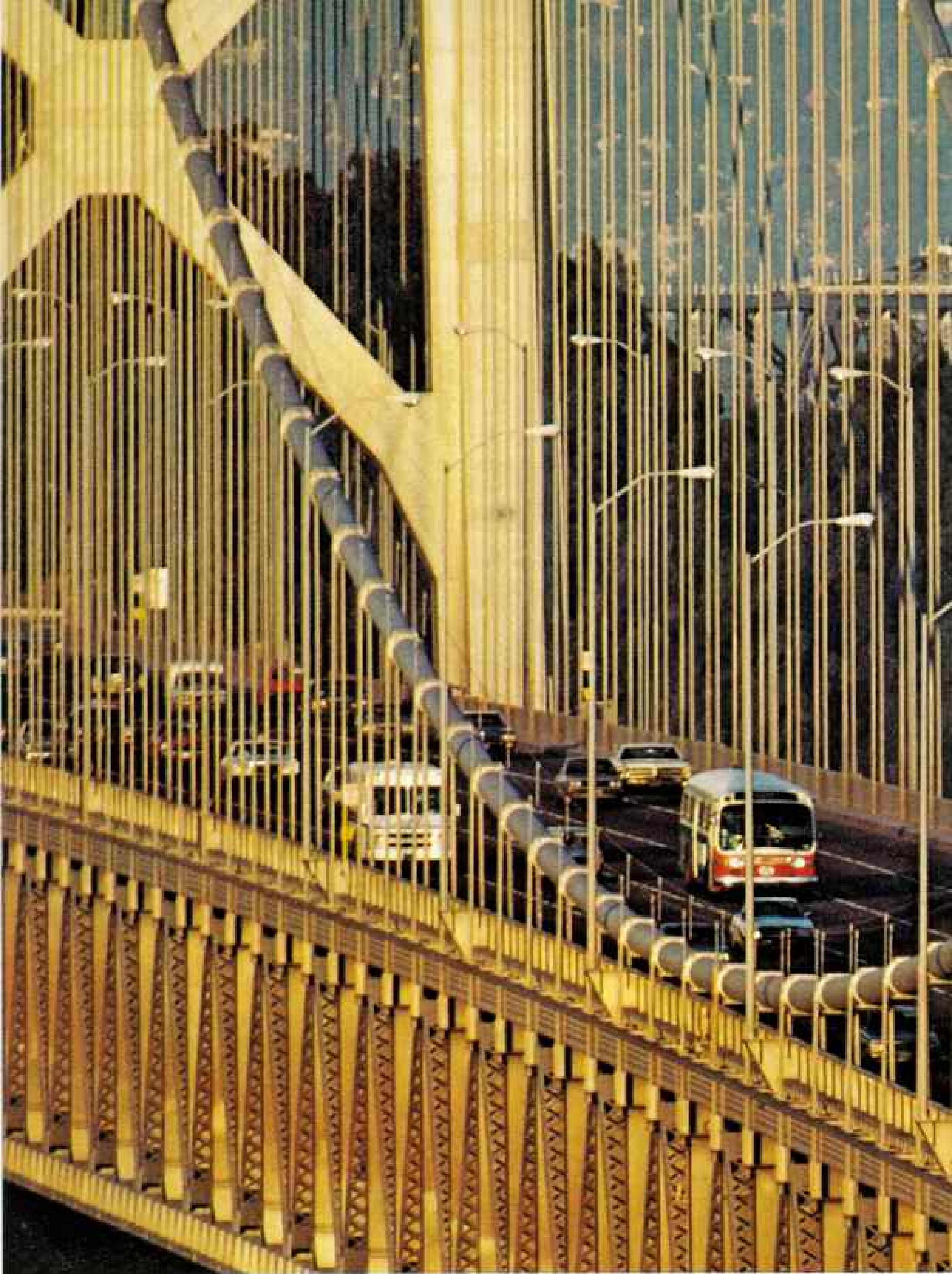
Caged in a forest of metal, traffic in the westbound lanes of the double-
