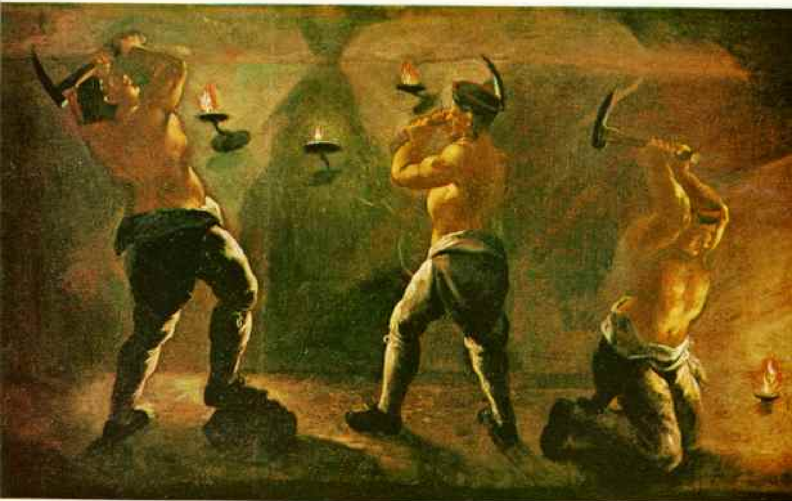
SALINENHERRN TUNEL, HALLSTATT, AUSTRIA
