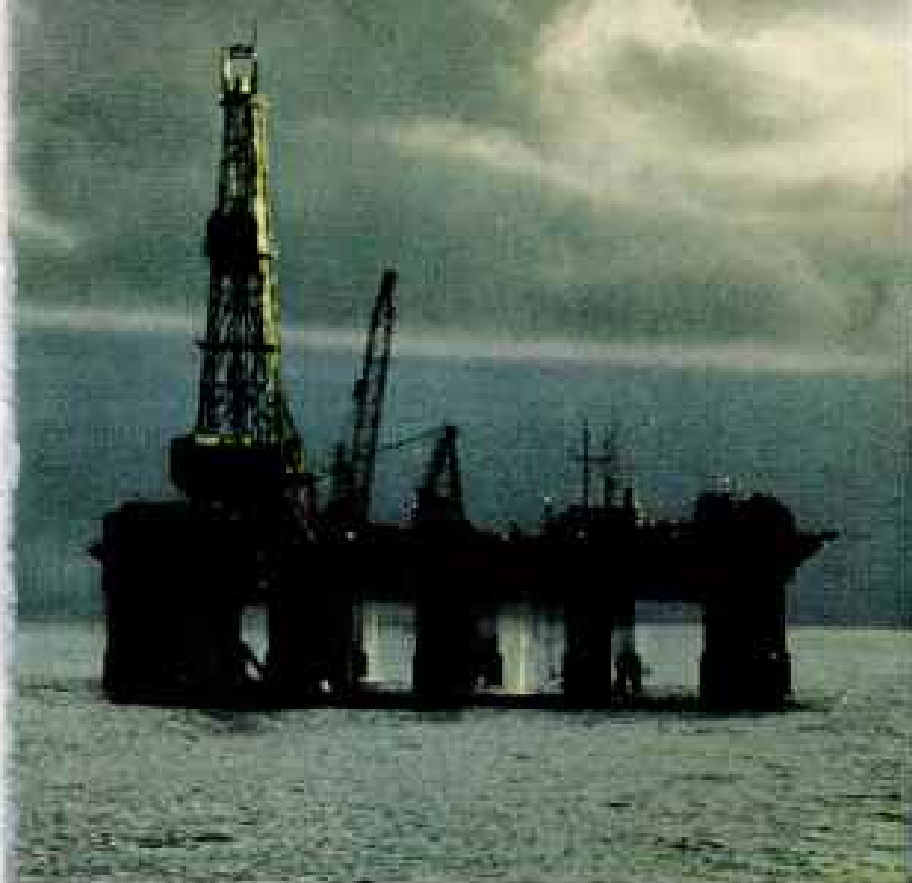
Exxon is looking for oil on land and off the coasts of more than 40 countries around the world. This platform is located in the North Sea where frequent storms bring 75-mile-an-hour winds and 65-foot waves.
