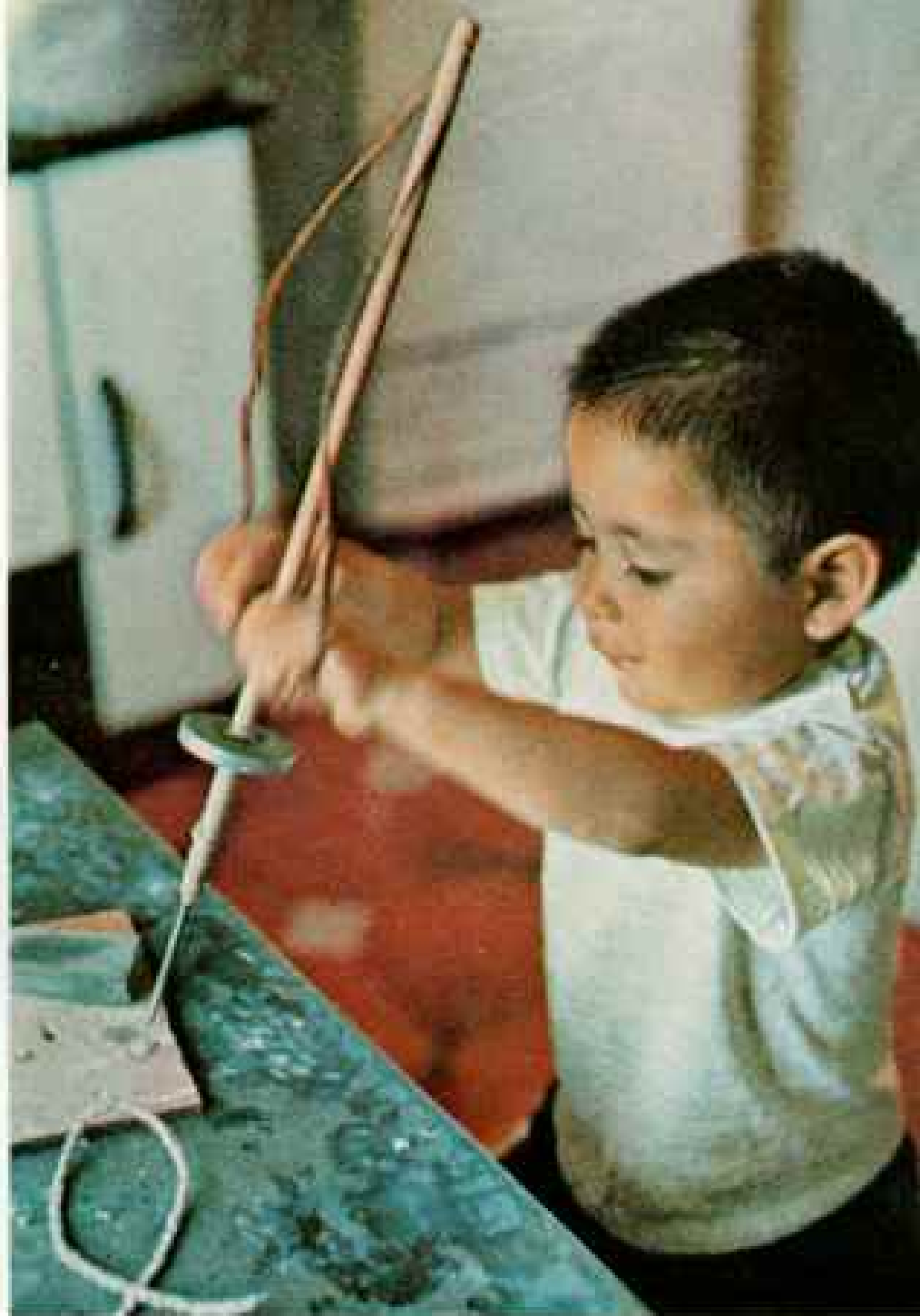
Junior bead maker of Santo Domingo bores shells with a hand drill whirled by thongs.
