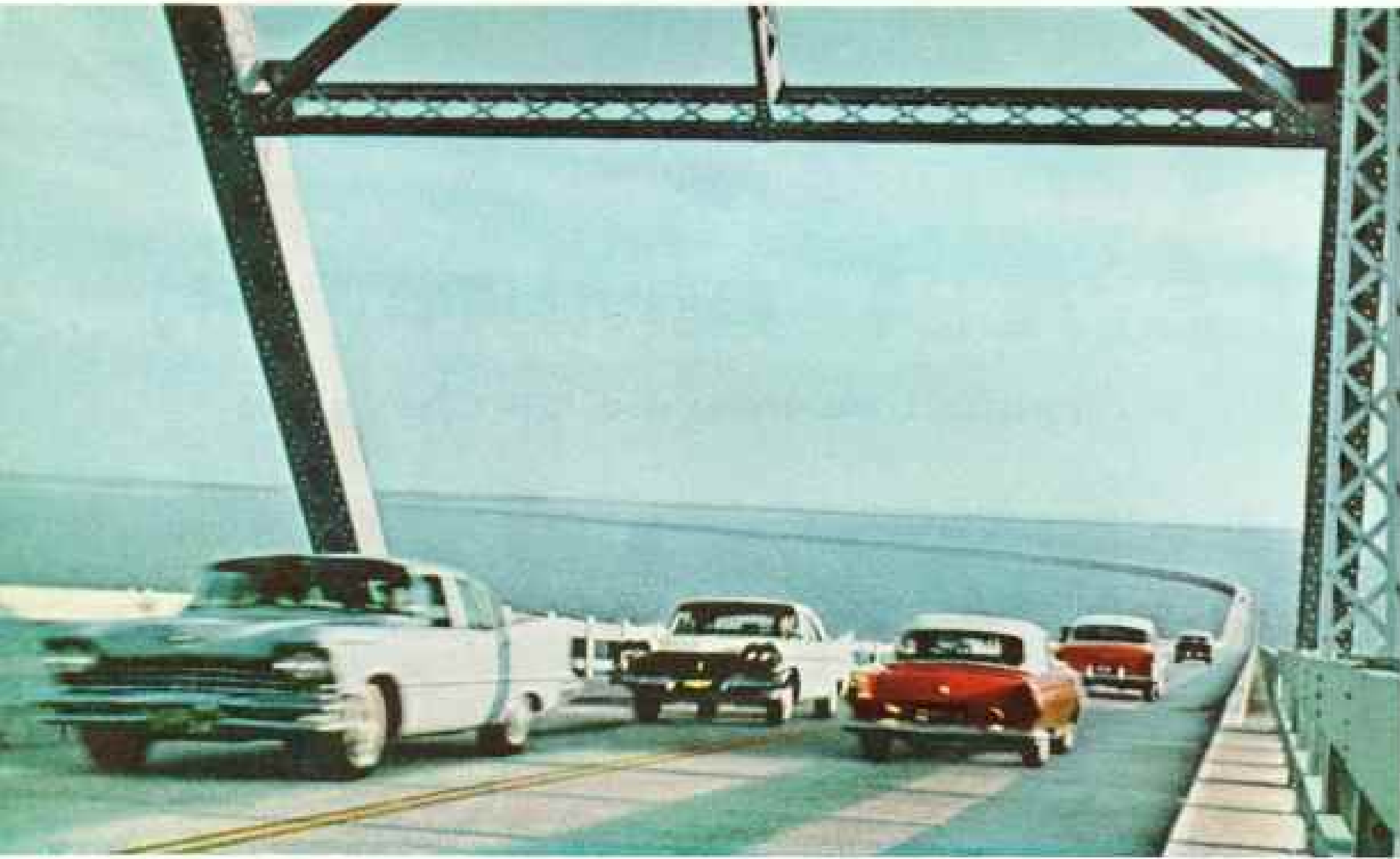
Florida's 15-mile "Sunshine Skyway" over Lower Tampa Bay.
