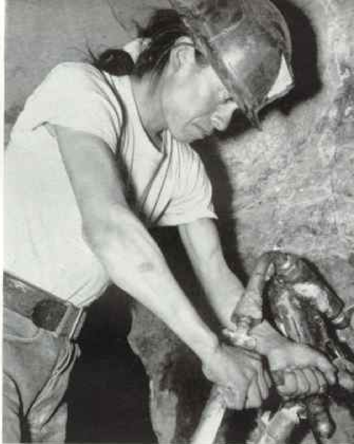
Helmeted, long-haired Navajo repairs his jackhammer in a Monument Valley uranium mine.
