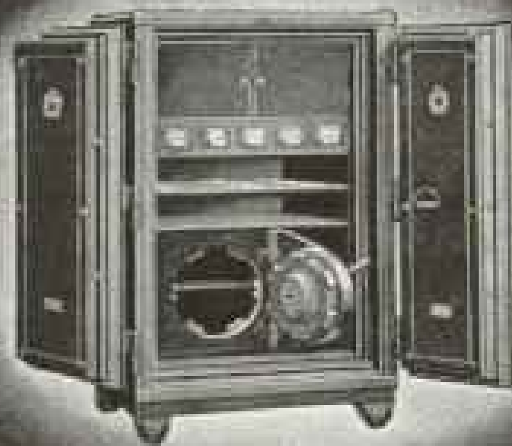
Mosler "A" Label Safe with burglary resistive chest for dual protection against fire and burglary.
