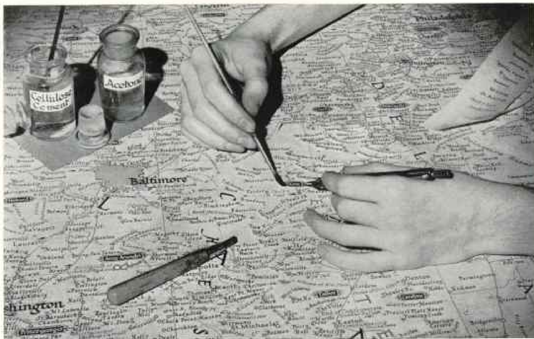
Each Name on a Geographic Map Is a Tiny Photographic Print from Hand Lettering
