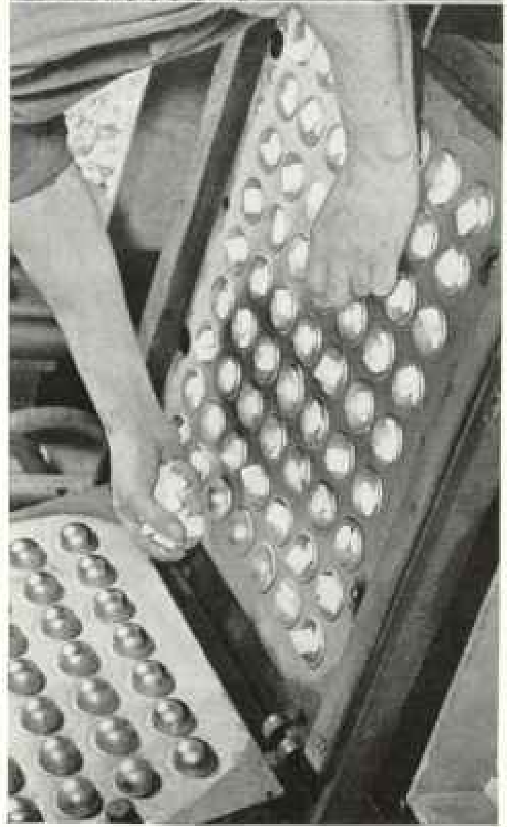
RUBBER BLOCKS MARK THE BIRTH OF A GOLF BALL A pill mold presses the cubes into spheres (page 191).
