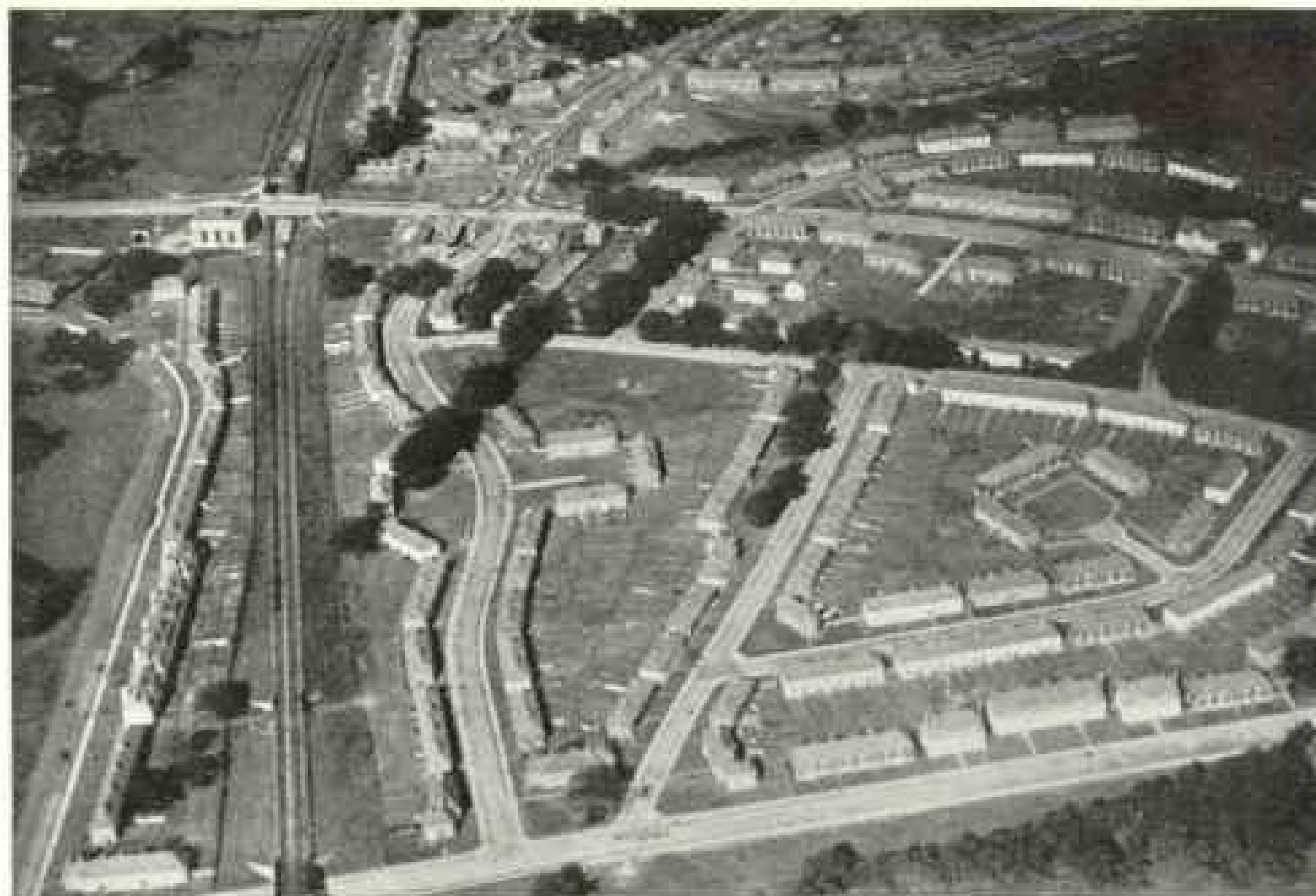
Photograph by Aerofilm
