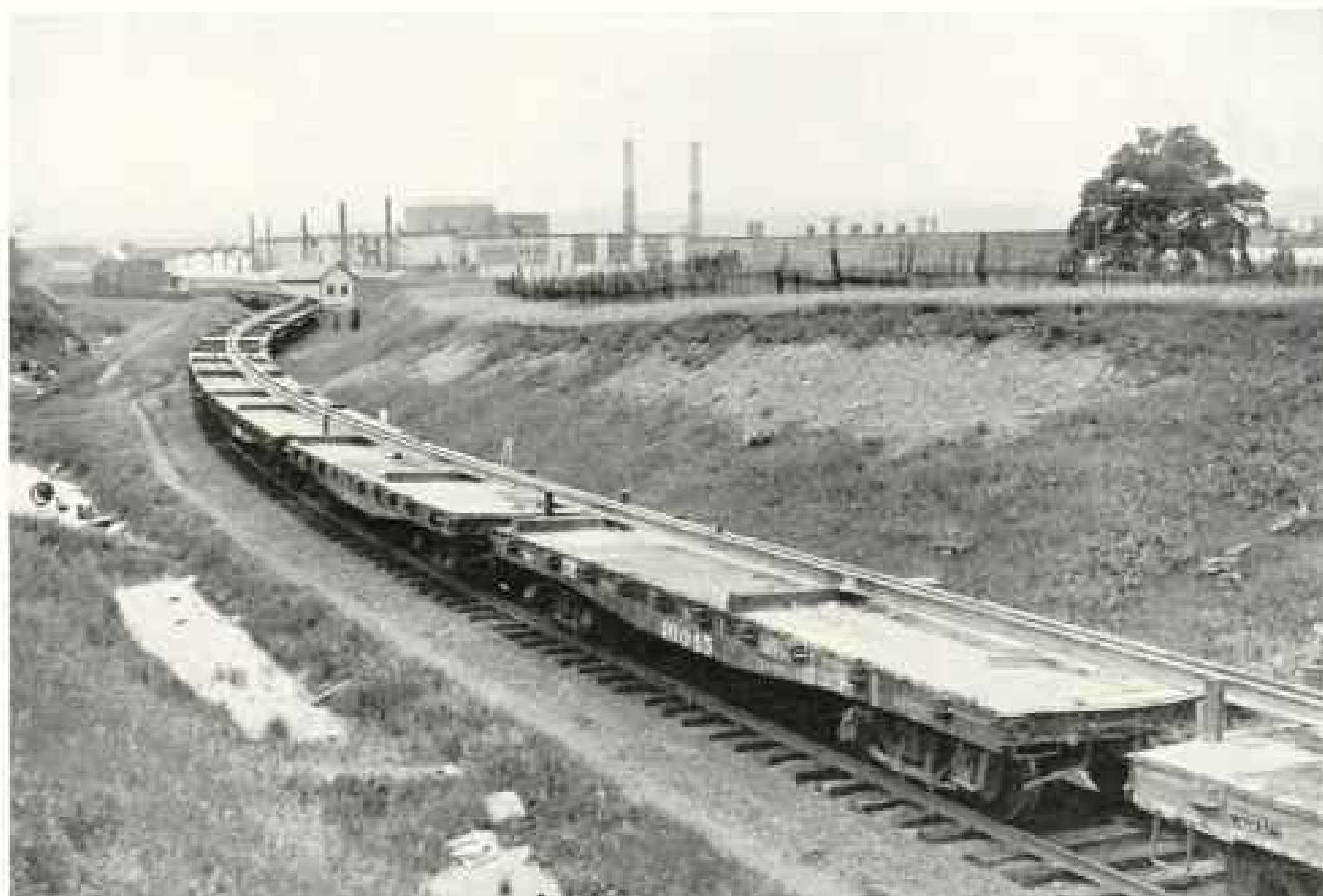
Photograph from W. W. Bates
