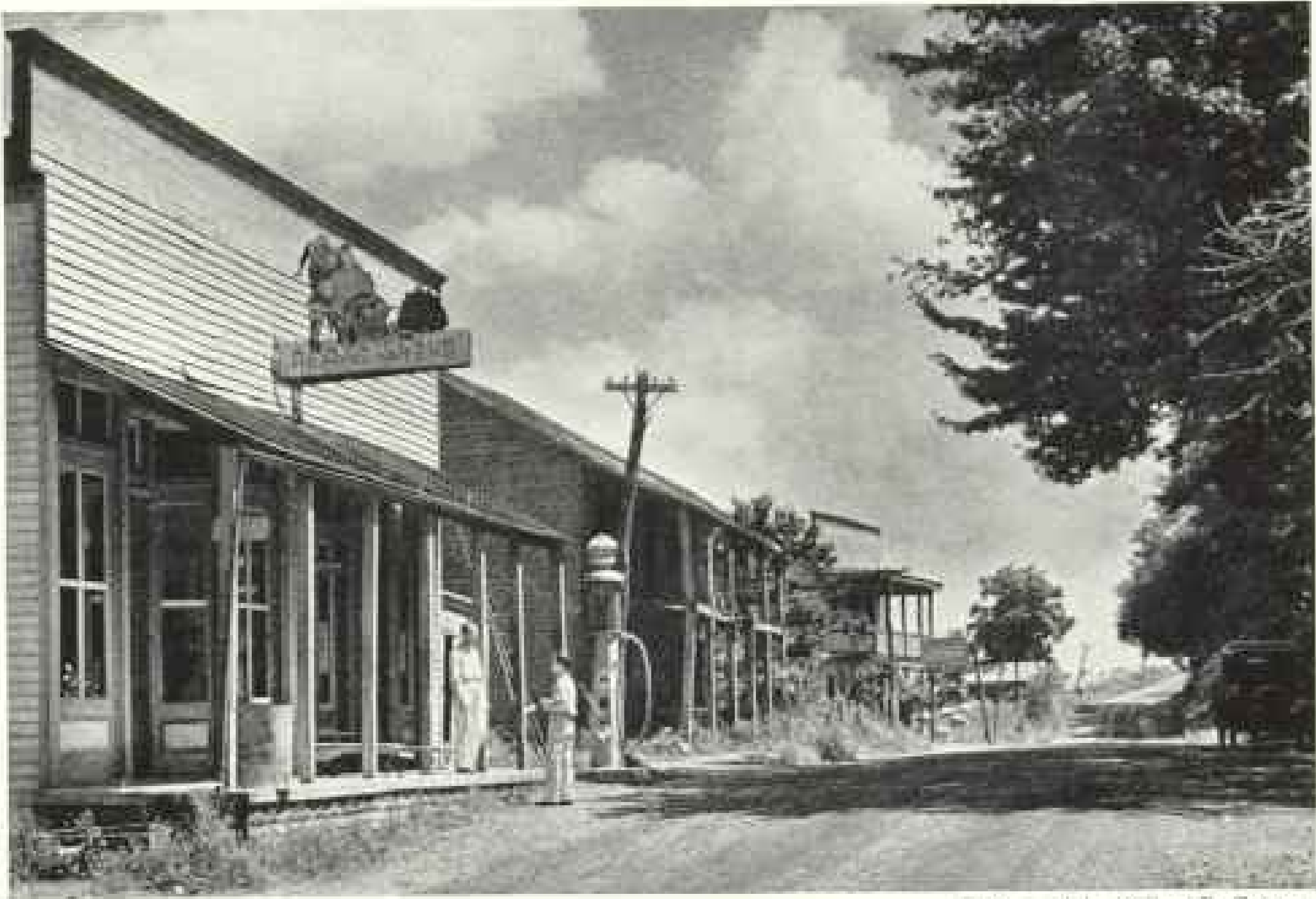
Photograph by Willard R. Culver
