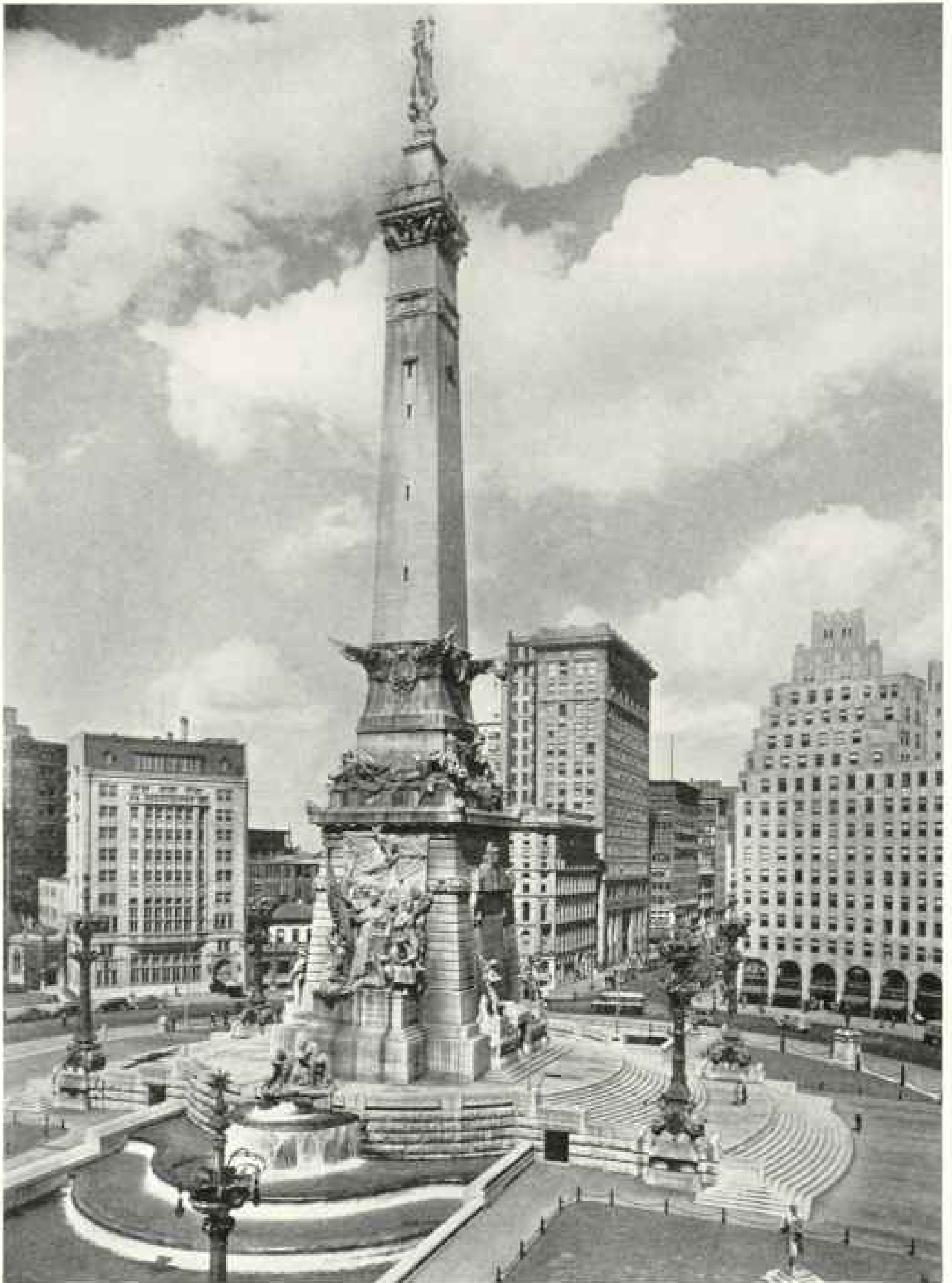
Photograph by Willard R. Culver
