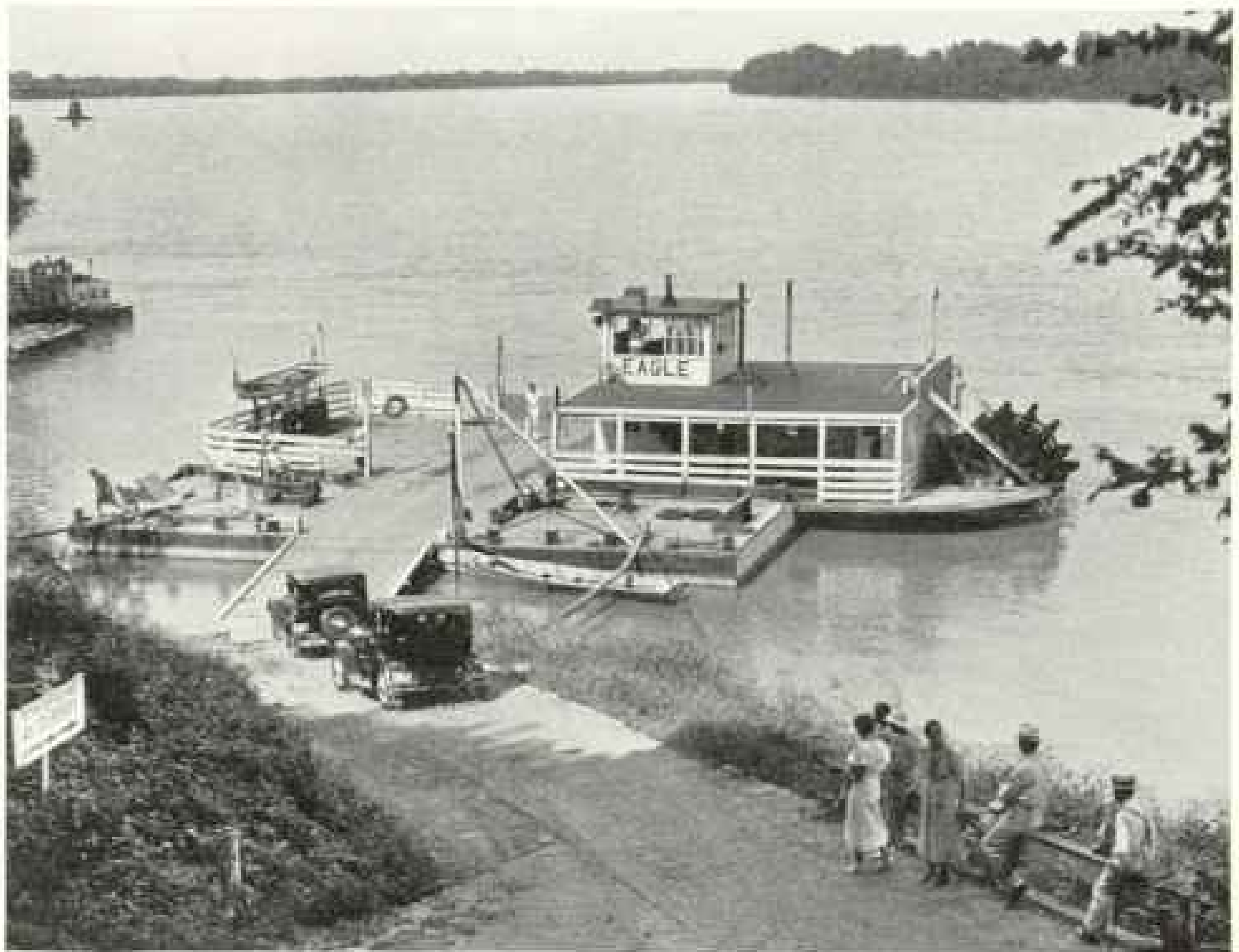
Photograph by Willard R. Culver
