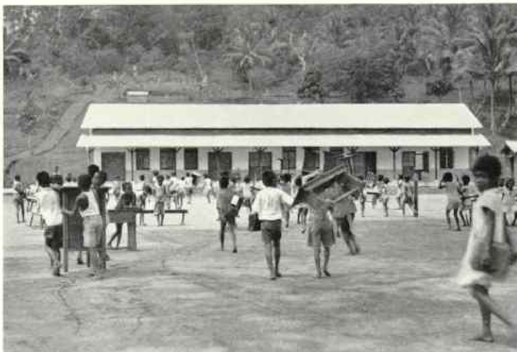
A NEW CONCRETE SCHOOLHOUSE OPENS IN A PALAU JUNGLE VILLAGE Students are busy carrying desks and benches from the old one in a native bathhouse.
