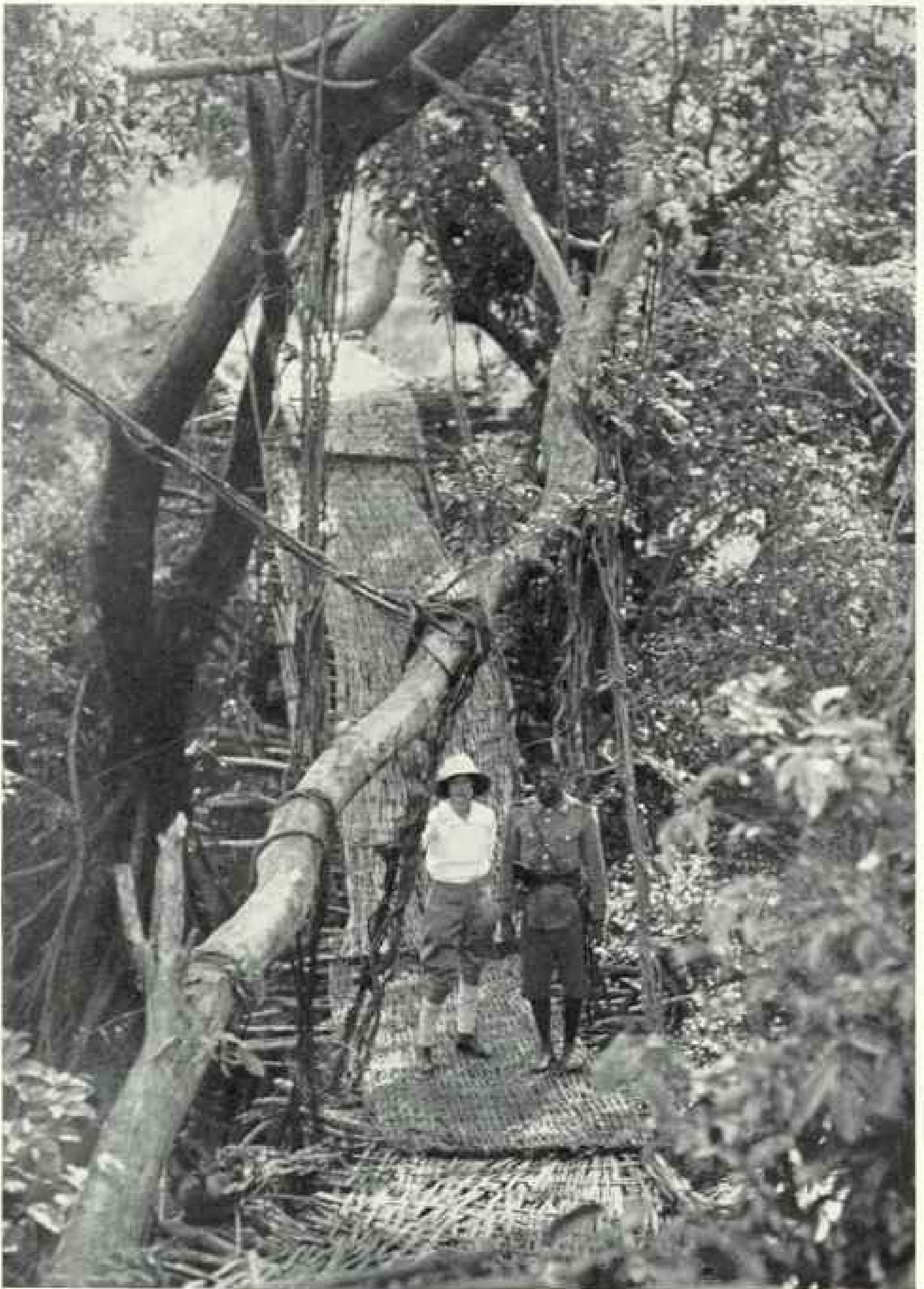
NATIVES USED THE MATERIAL AT HAND TO BUILD A SERVICEABLE BRIDGE
