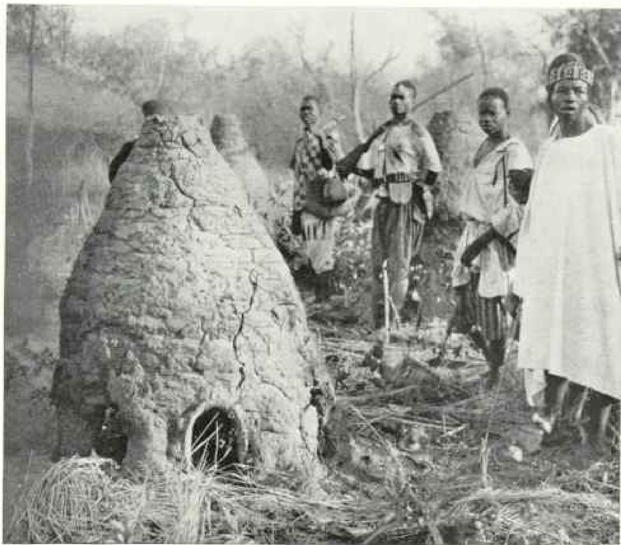
NATIVE ORE IS SMELTED IN THESE BLAST FURNACES
