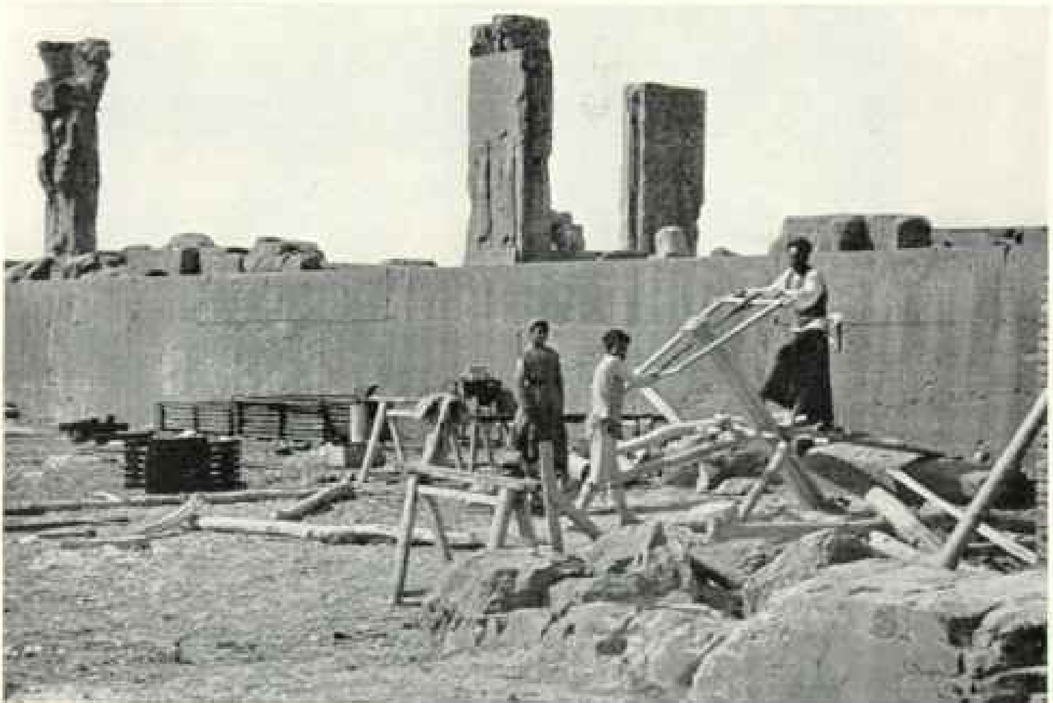
WITH A RIPSAW WORKMEN MAKE BOARDS TO REPAIR AN ANCIENT HAREM
