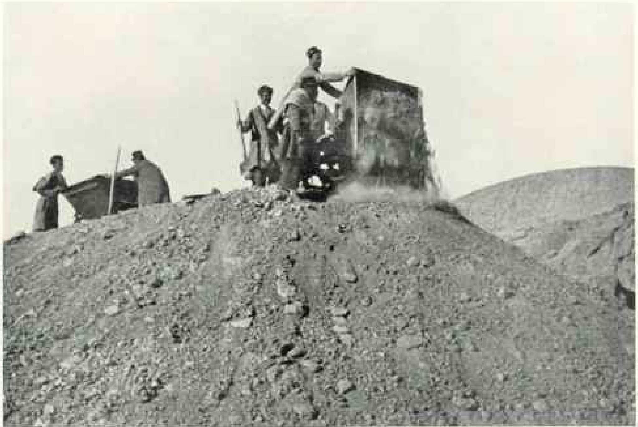
DUMPING WASTE REMOVED FROM THE RUINS
