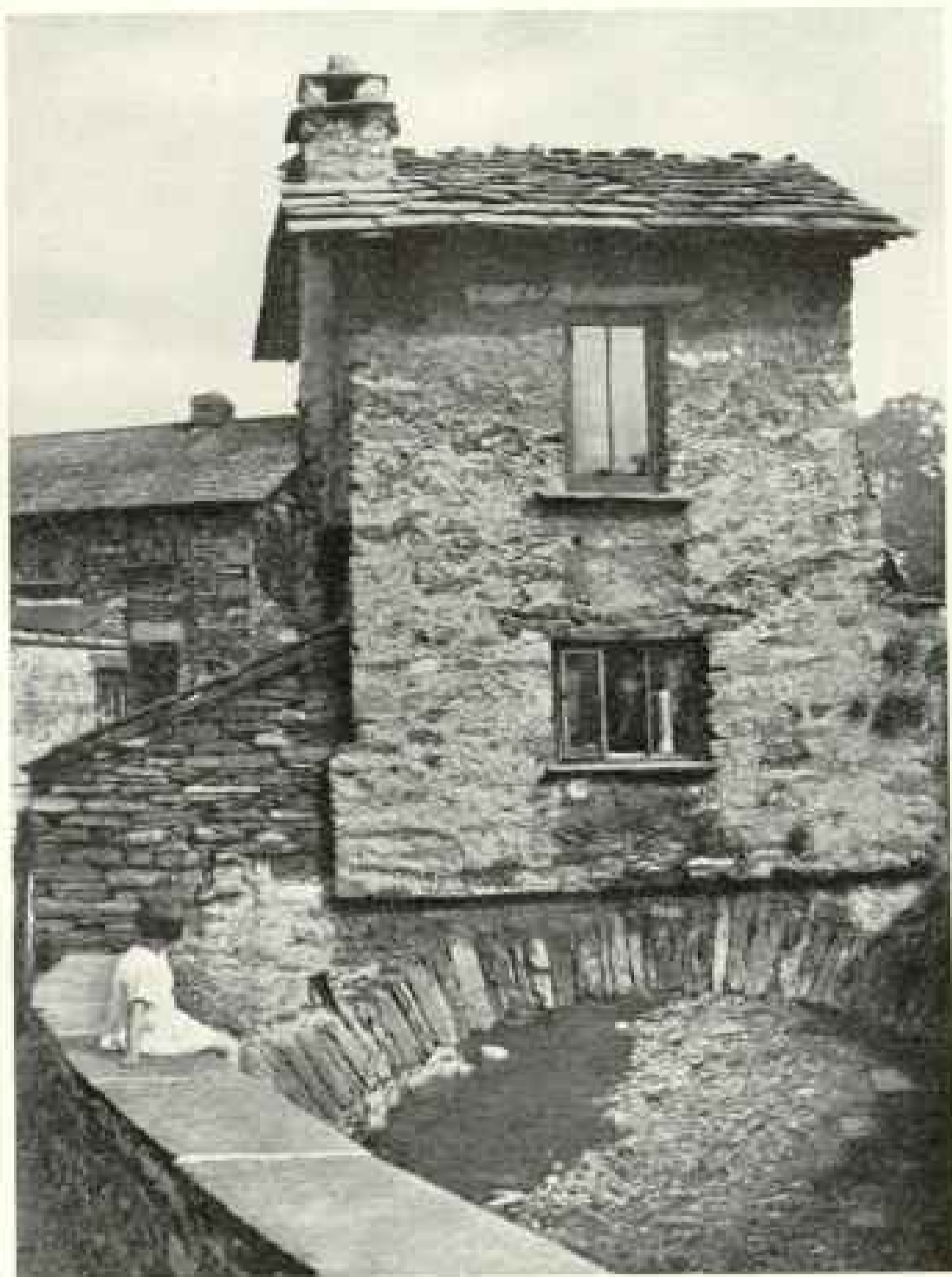
BRIDGE HOUSE CATCHES EVERY PASSING EYE
