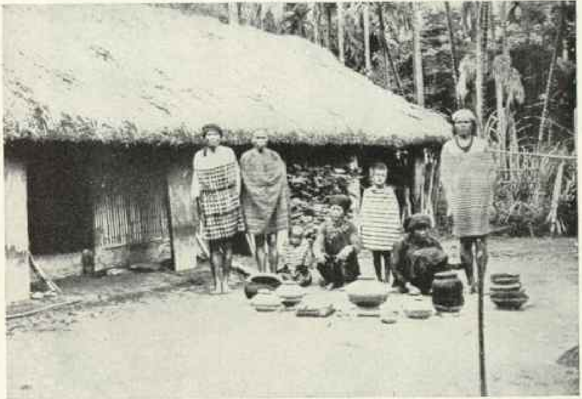
A THATCHED-ROOF TYPE OF SAVAGE DWELLING These natives are displaying some of their hand-made pottery.
