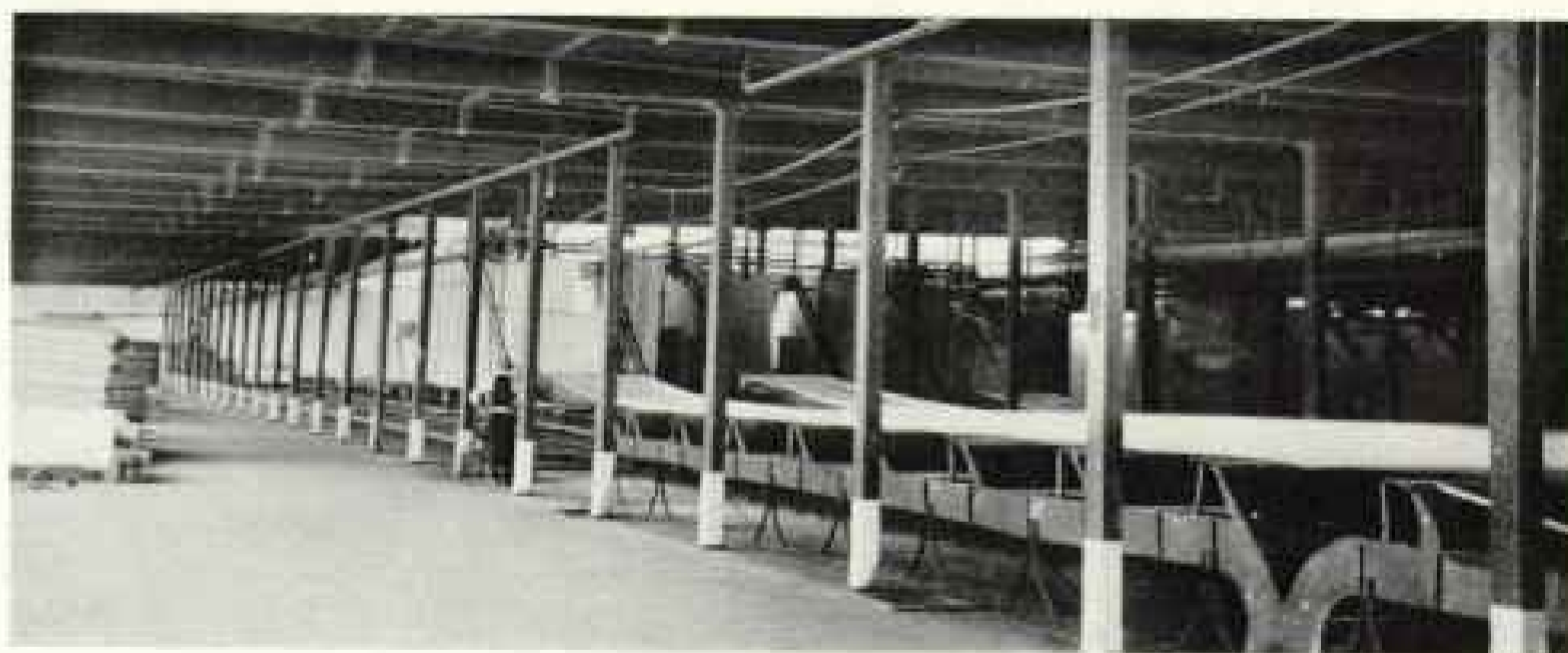
THE DRYING-ROOM IN THE COATING MILL AT LAWRENCE, MASS.
