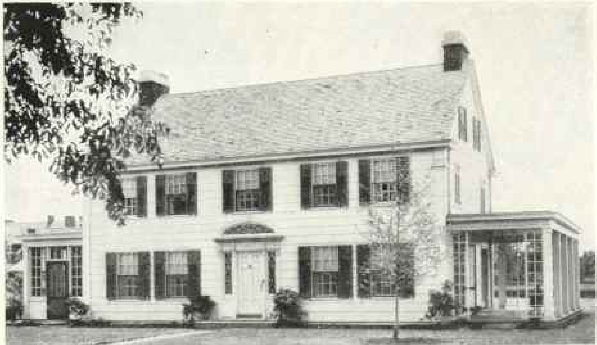
House of F. P. Clark, Esq., Garden City, New York. Architect, Arthur Embury II, New York City.
