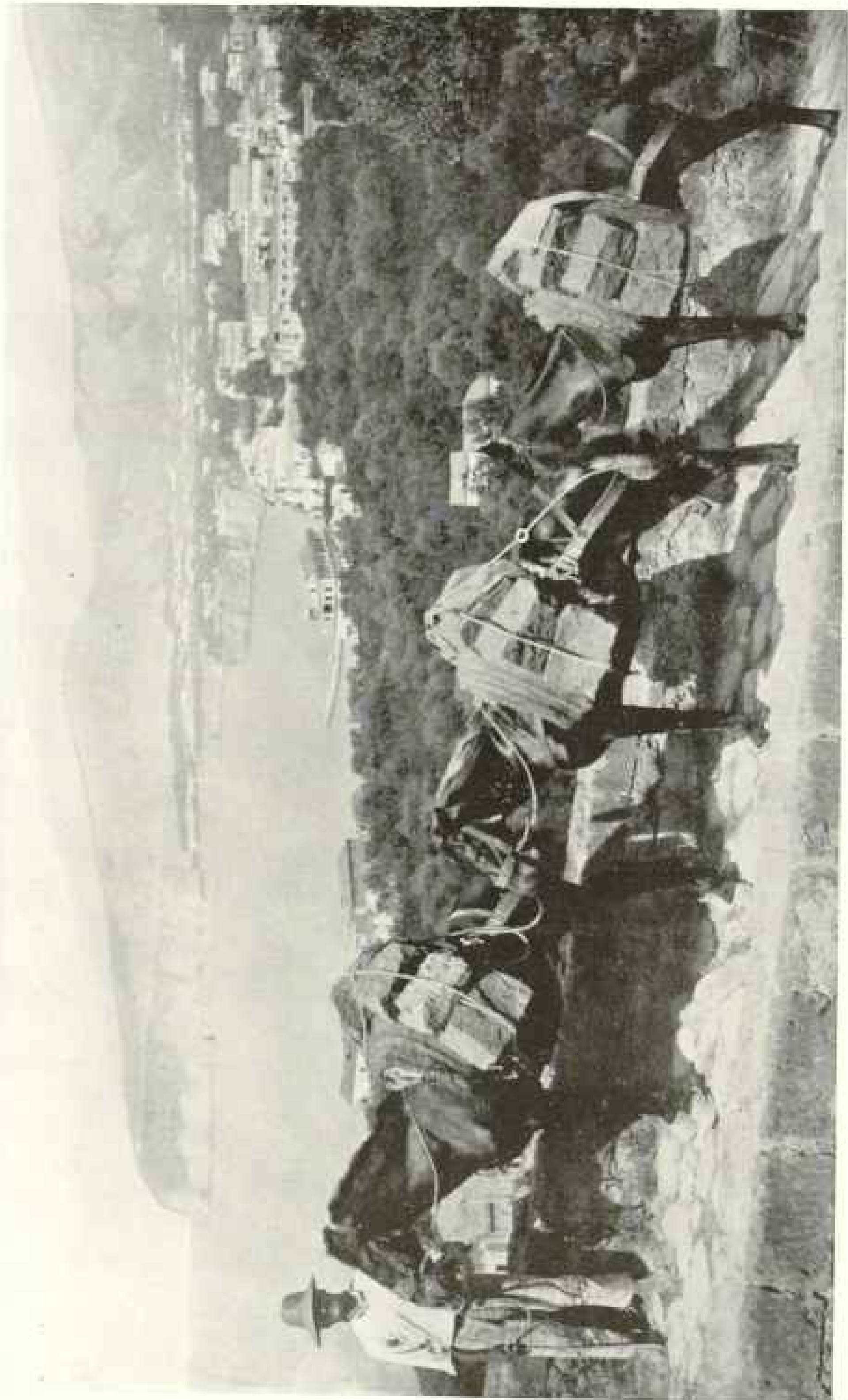
SORRENTINE MOTOR TRUCKS: MANY OF THE EDIFICES ERECTED ON THE CLIFF AT SORRENTO WERE BUILT WITH BLOCKS OF STONE BROUGHT UP ON THE BACKS OF MULES
