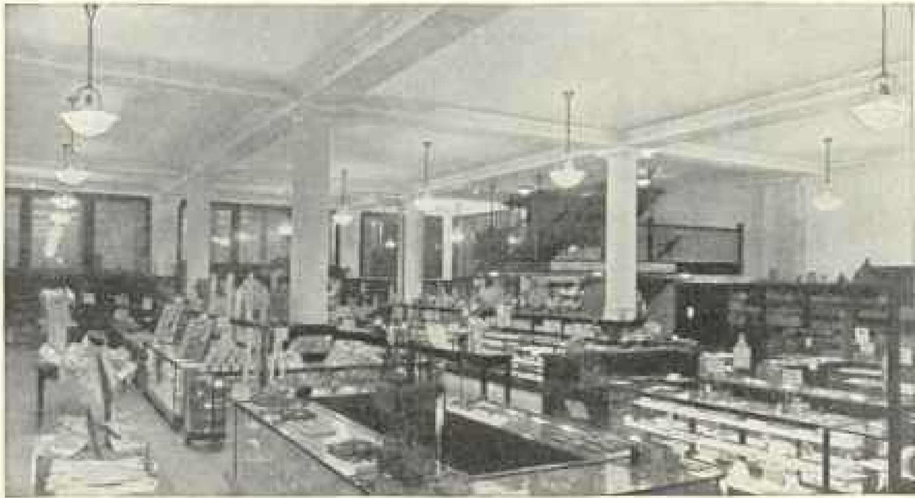
H. Leh and Company's store, Allentown, Pa.—Alba-lighted throughout.
