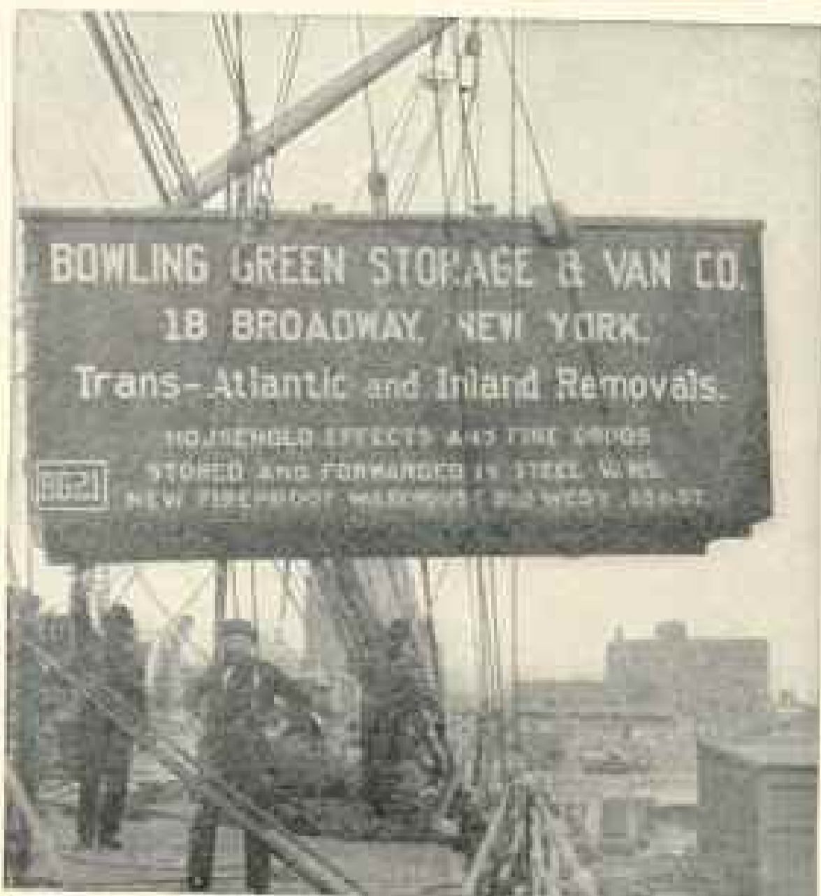
HOISTING LIFT-VAN ON BOARD STEAMSHIP
