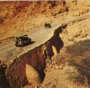
Roman bridge, still in use
