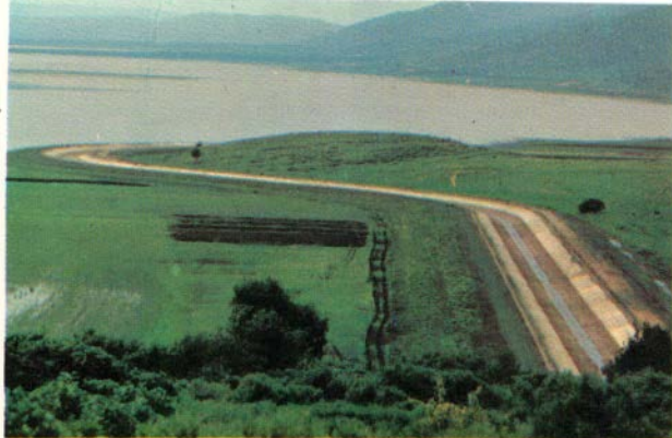
National Water Carrier from the Sea of Galilee to the Negev Desert
