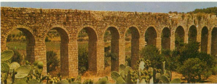
Turkish aqueduct in Naharia, north of Haifa
