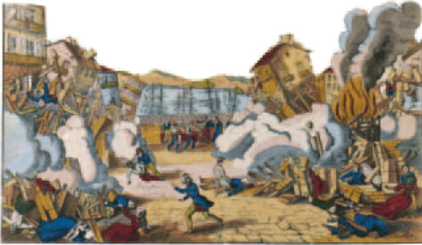
DEVASTATED IN A MINUTE The town of Pointe-à-Pitre on the Caribbean island of Guadeloupe was shaken by an earthquake of Richter magnitude 8 on February 8, 1843. Eyewitnesses said the shaking lasted for about a minute. This was long enough to reduce most of the buildings to ruins. A fire that followed torched what was left of the town.
