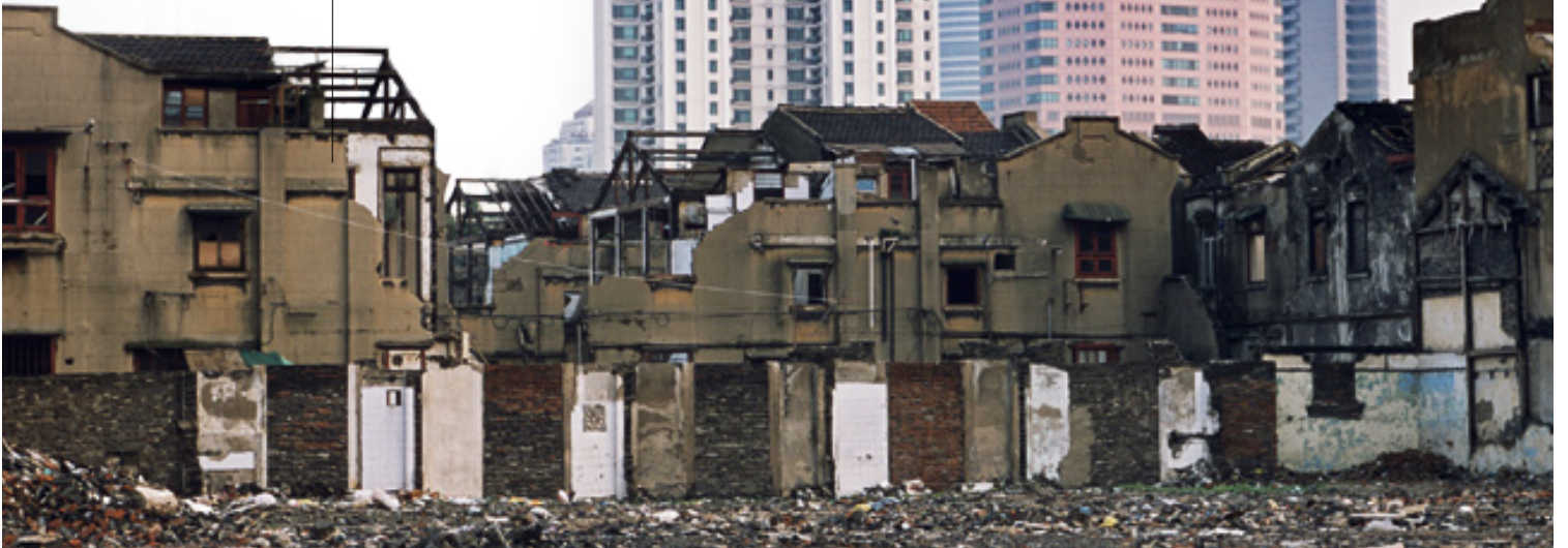
Old houses awaiting demolition
