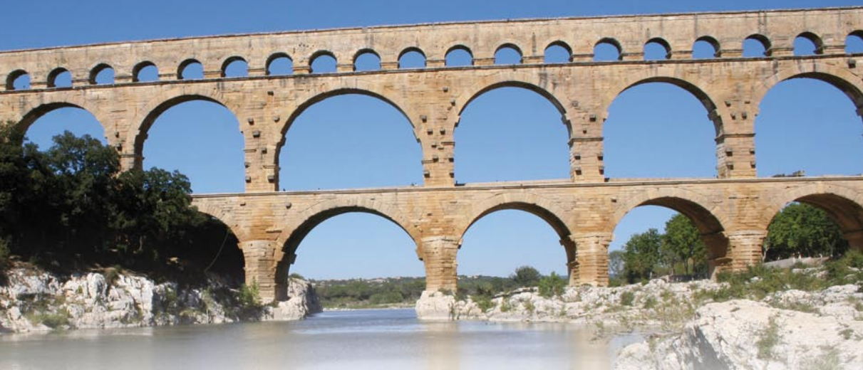
PONT DU GARD, A STONE AQUEDUCT IN SOUTHERN FRANCE
