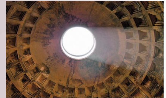
Concrete dome of the Pantheon, a temple in Rome
