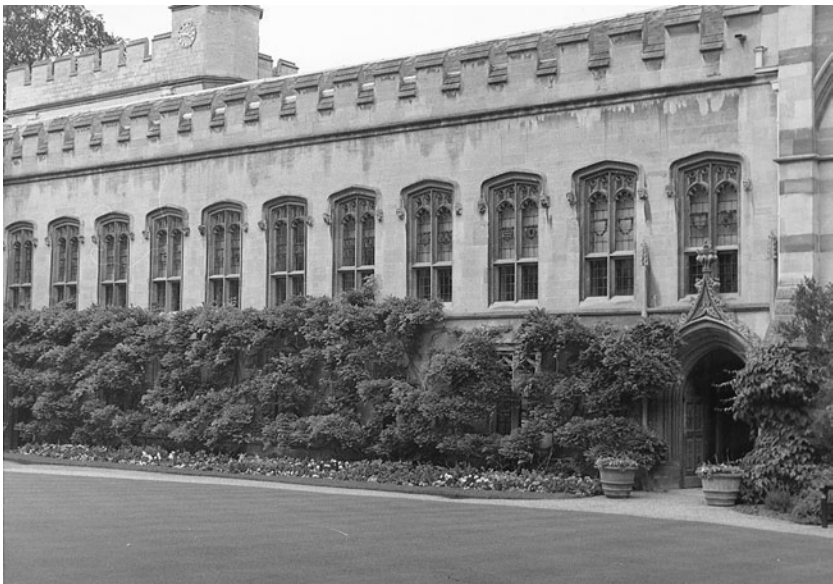
Figure 16 Balliol College, Oxford, from quad, north side, showing the elevation of the medieval library room. (Photo, Gameson)
