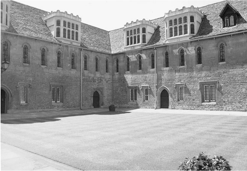
Figure 6 Merton College, Oxford, Mob Quad, north and east sides. The 'noua libraria' occupied the first floor of both ranges. (Photo, Gameson)
