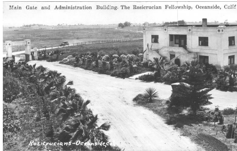
72. Main entrance with Administration Building.
