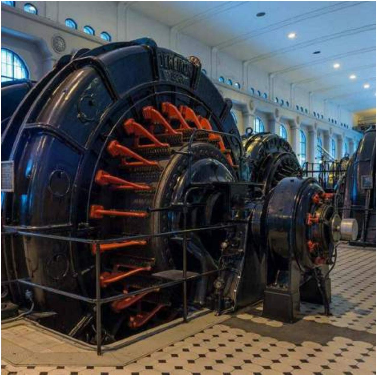
FIG. 10 — Turbines currently exposed at the Industrial Workers Museum built by the German engineering company Voith in Heidenheim and the Zürich firm A/G Escher Wyss for the Norsk-Hydro Works near Rjukan, the only industrial plant under German control capable of producing heavy water (deuterium oxide, D 2 O) in significant quantities.
