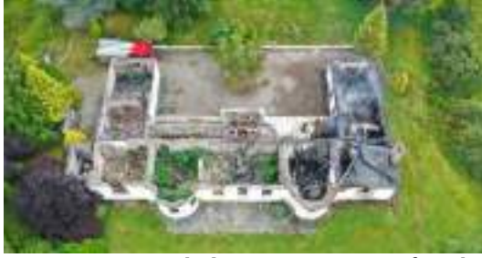
FIG. 46 – Boleskine House ruins after the first fire shows there was extensive damage (photo courtesy of Infowars).
