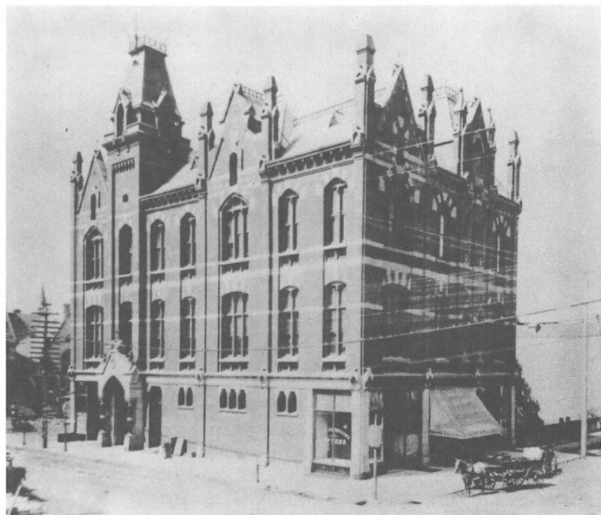
4. Oakland Masonic Temple, exterior
