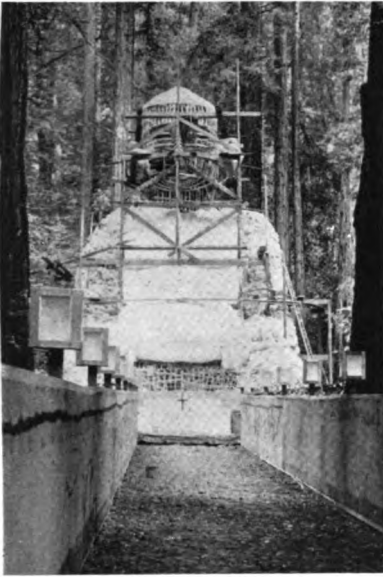
CONSTRUCTING THE DAI-BUTSU (1892)
