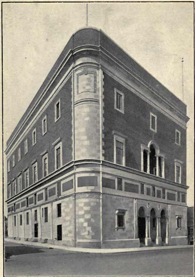
Masonic Temple, Yonge Street and Davenport Road, in which St. Andrew's Lodge met in 1922.
