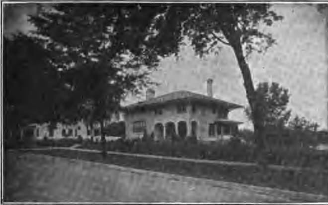
Front View of Building
