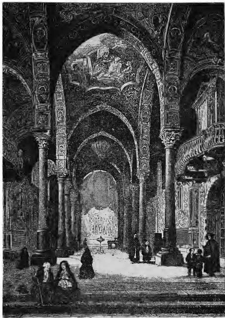
Interior of Church of St. Simon, at Palermo.
