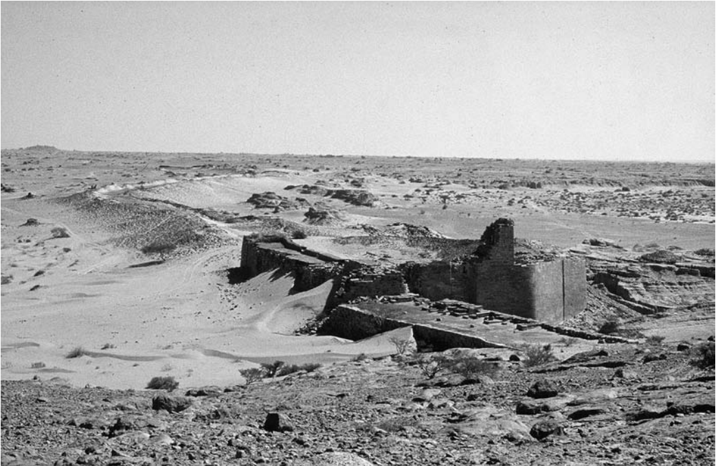
[111] The dam of the southern Arabian city of Ma'rib (Marib): northern sluice and canal. Photograph courtesy of Christian Robin.
