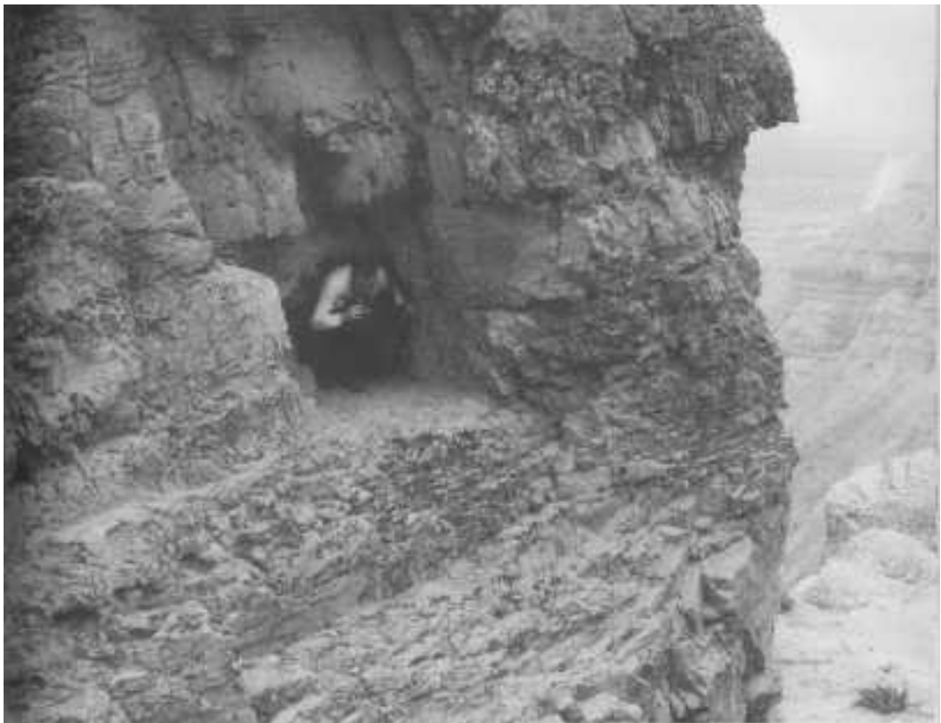
34 The water supply to Qumran depended upon this water tunnel carved through solid rock
