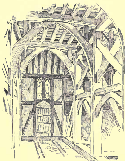
TIMBER WORK OF TOWER OF MARGARETTING CHURCH.
