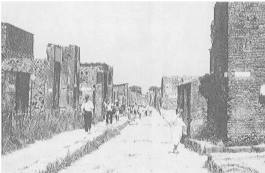
Figure 12.1 Street with raised pavement to the side, and 'stepping stones' for crossing to the other side.
