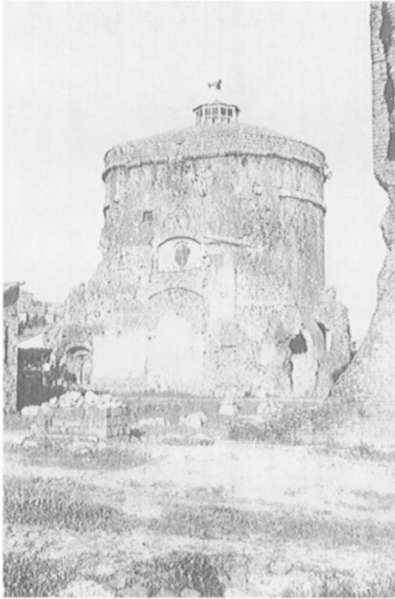
Figure 8.6 The north wing of the great Precinct of Isis, built of mortared red brick and still intact, functioning as a mosque.
