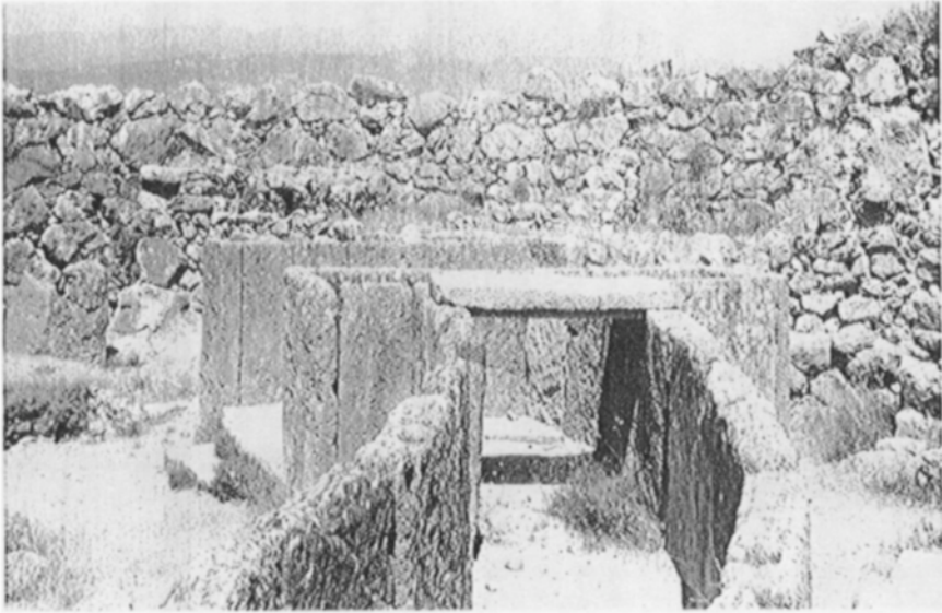
Figure 3.4 The wall, comprising two lines of upright slabs with slabs across them, around Grave Circle A.
