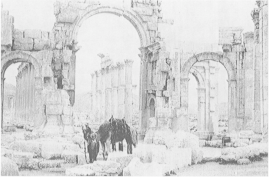
Figure 14.4 Triangular-plan triple archway, masking the change of alignment in the colonnaded streets.
