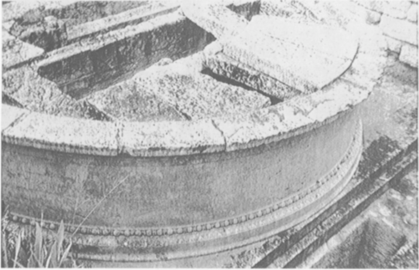
Figure 10.4 The Tomb of Battos in the Agora. A circular monument, with arrangements for offerings to the founder-hero of the city. The details (particularly the mouldings at the base of the circular structure) suggest that what survives was not built until the fourth century BC, presumably over an existing shrine.
