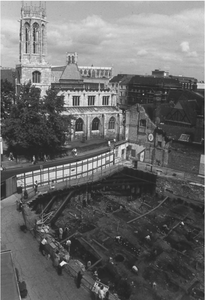
10. Excavations in progress at Coppergate, York
