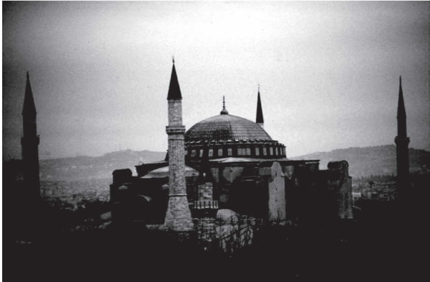
Plate 18.2 Hagia Sophia, Constantinople, 532–7. Exterior view from the south (Photo: Sasha Grishin)
