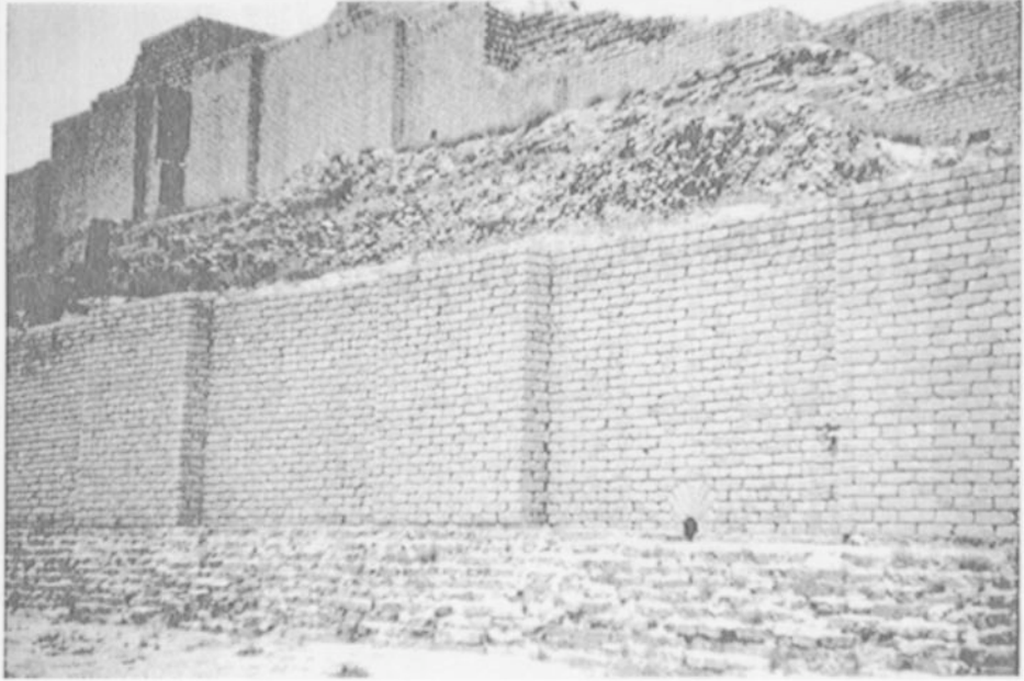
Buttresses on the retaining walls of the ziggurat at Choga Zanbil (restored)
