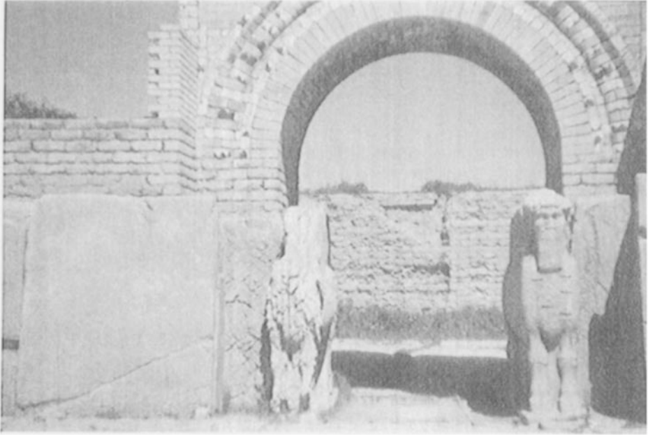
Palace of Nimrud: gate (restored)
