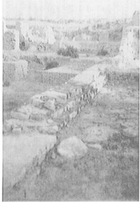
Baked bricks set in bitumen (Babylon, palace of Nebukadrezzar)
