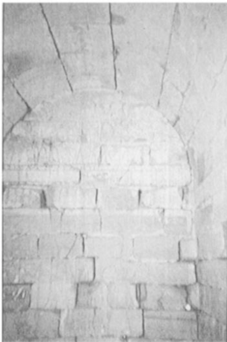
Barrel vault at Deir-el-Medineh, Ptolemaic temple
