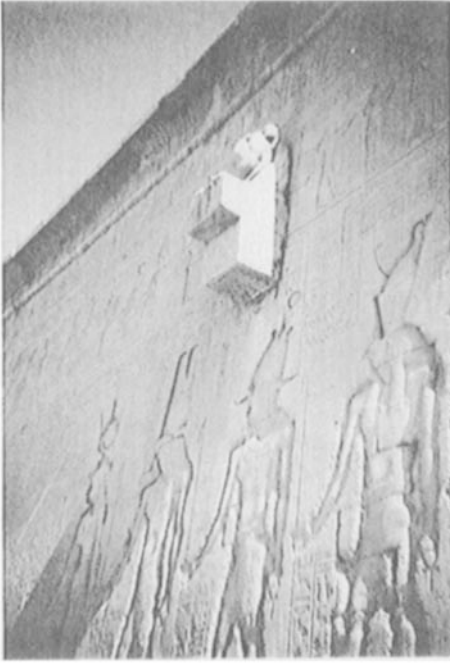
Roof drainage by lion-shaped spout, Dendera, Egypt (Graeco-Roman period)
