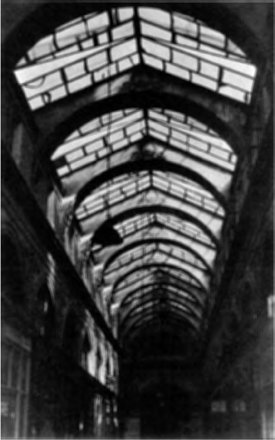
Glass roof and iron girders, Passage Vivienne. Photographer unknown. Collection of Johann Friedrich Geist; courtesy Prestel Verlag, Munich. See A1a,2.
