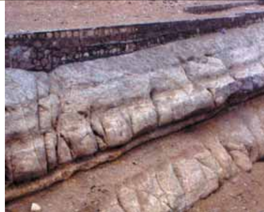
Telltale water weathering in Sphinx enclosure
