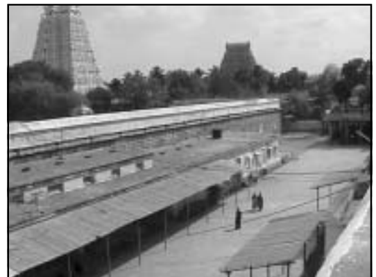
According to traditional sources, the Ranganatha temple's third boundary wall, shown here, was constructed about five thousand years ago.
