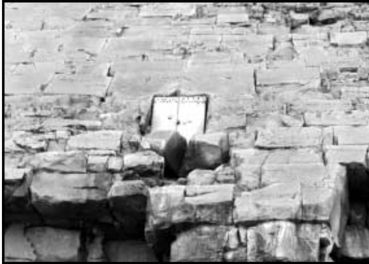
Repairs to Bent Pyramid
