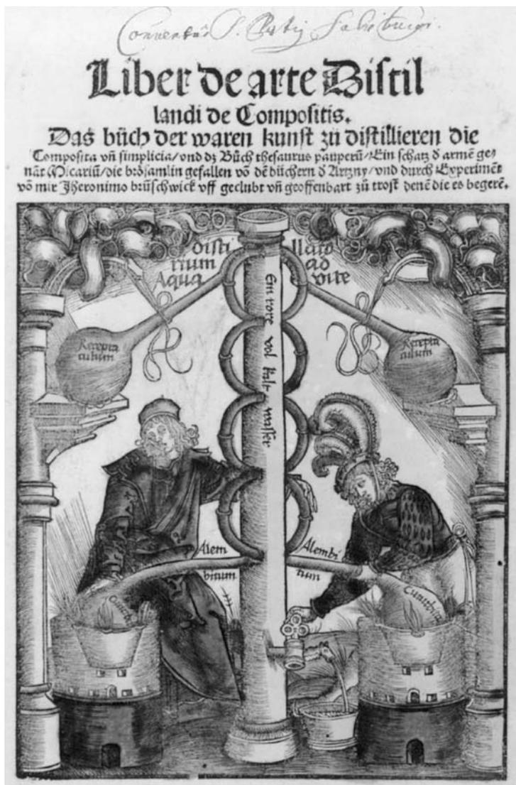
**FIGURE 99.** ■ Title page (hand-colored; see color plates) from *Liber de Arte Distillandi* (Hieronymus Brunschwig, 1512), depicting a double-still in which the central tower contains cooling water that is continuously replenished. Come to think of it, this apparatus evokes an image of the caduceus: two serpents entwined about the staff of Hermes where the loops symbolize “couplings.” (From the Othmer Library, CHF.)
