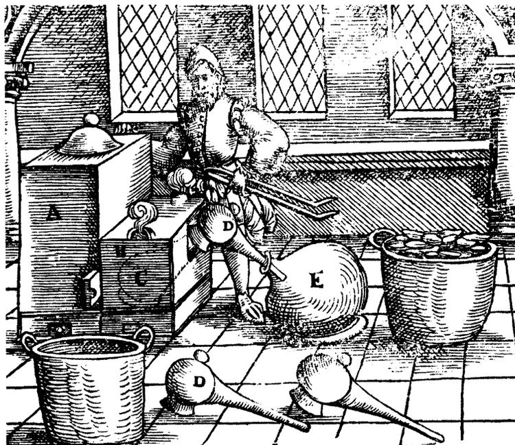
**FIGURE 12.** ■ Distillation of *aqua regia* (3:1 HCl/HNO<sub>3</sub>) (Ercker, see Figure 5). This “kingly water” is capable of dissolving gold. (See essay in Section IX “The Chemistry of Gold is Noble But Not Simple.”)
