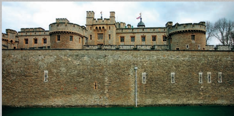
The White Tower that forms the keep to the Tower of London was built by William the Conqueror between 1078 and 1090. It is set within two parallel rings of defensive walls and a moat. Note the arrow slits in the outer wall, which are characteristic of Norman architecture.
