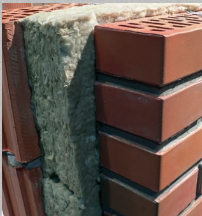
Picture are a steel-frame structure (left) under construction, and a load-bearing brick wall (above) with insulated cavity.
