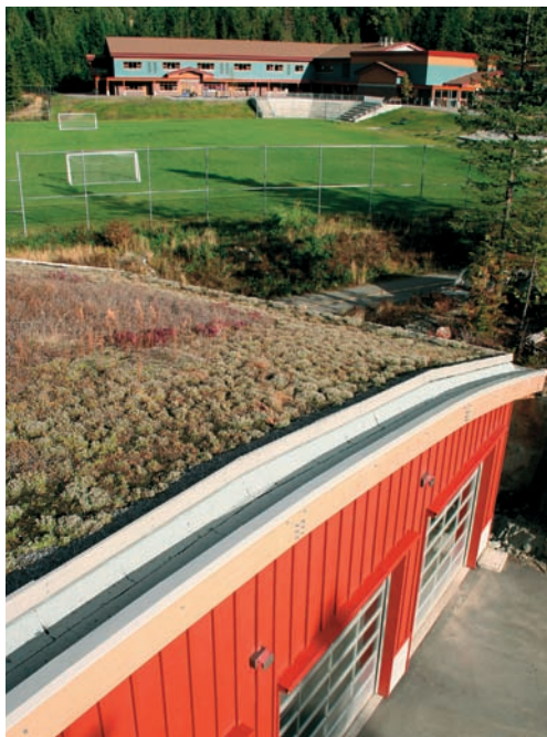
The Spring Creek Fire Station in Whistler, Canada (left) has a number of energy-efficient features including air recovery units, efficient heating systems and a green roof, which reflects solar gain and acts to insulate the building.
