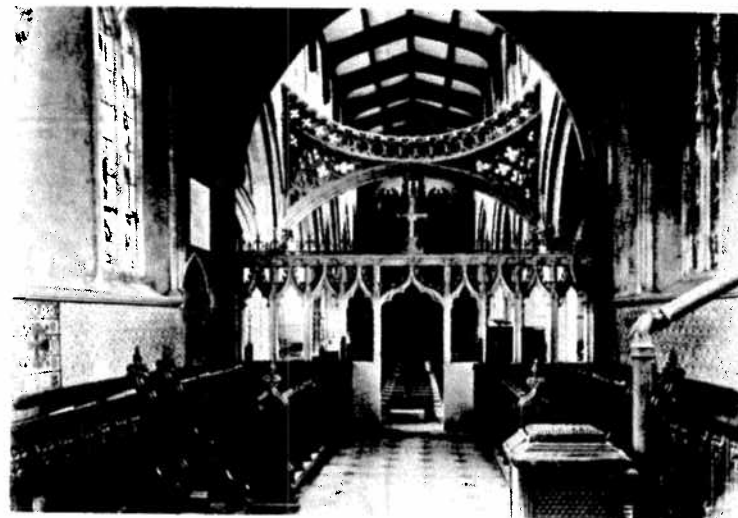
PLATE 6 St Mary Finedon, Northants, strainer arch
