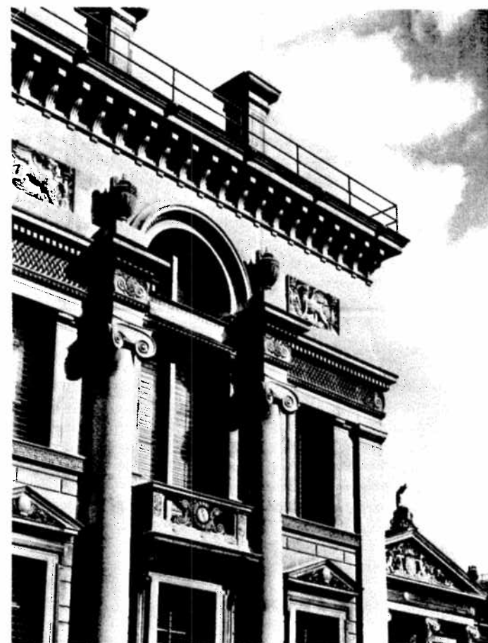
PLATE 59 C. R. Cockerell: Ashmolean Museum, Oxford, detail of façade
