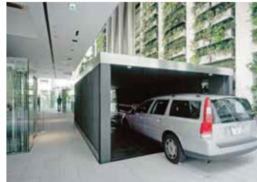
Below A car elevator emerges from the ground floor to take cars to an underground parking lot, a luxury in this very tight site.
